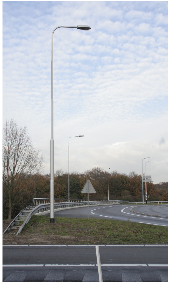
Example of a passive safe pole with a non-standard collision angle.
