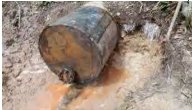
Photo 6: Detail of the pipe after being re-sealed.
